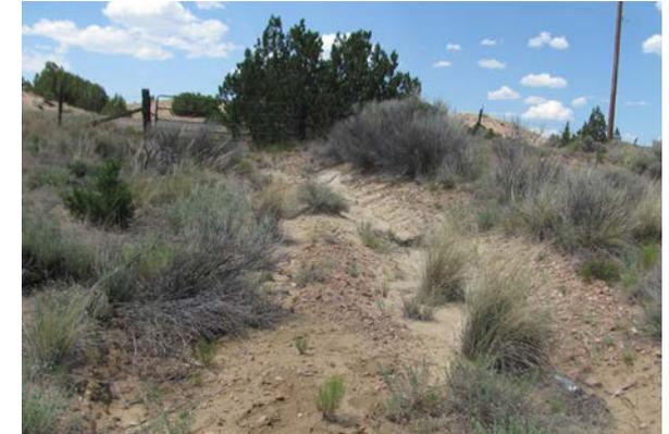
Photo 15. Eroded access road to EAWSD well.
